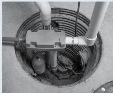
Your "friend" typically sits in the lowest level of your home and is designed to remove excess water after heavy rains and snow melts. The sump pump moves water from the pit to a location away
