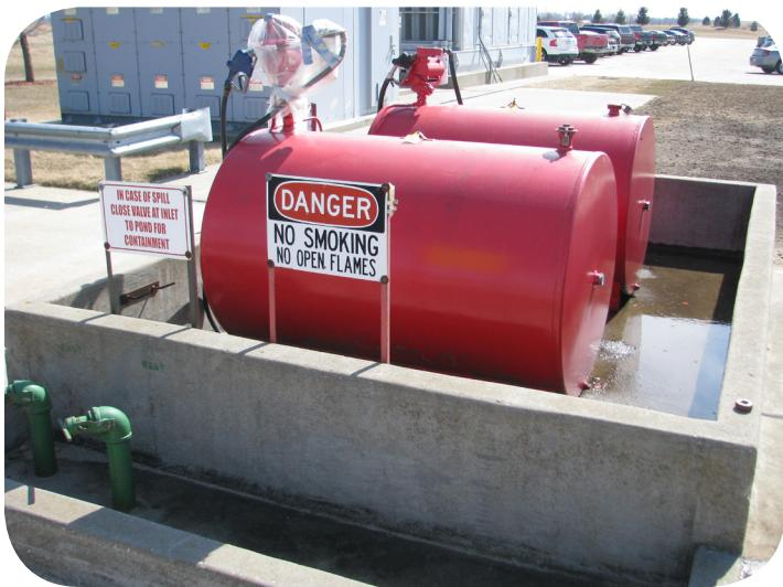
Storage tanks and their accessories shall be inspected and maintained according to manufacturer's guidelines or applicable standards. Every aboveground tank shall have an emergency relief venting device to relieve excessive internal pressure caused by an exposure fire.
